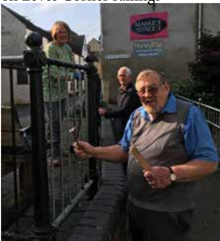
committee members get to work on Lèves Corner railings
